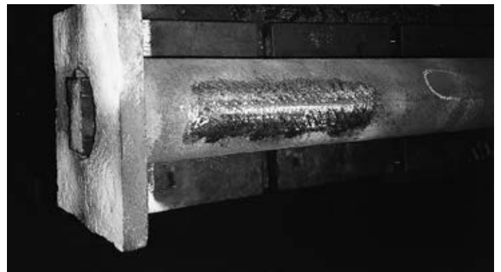
Below: Bellway Home support columns showing the removal and replacement of damaged sections in the workshop.
