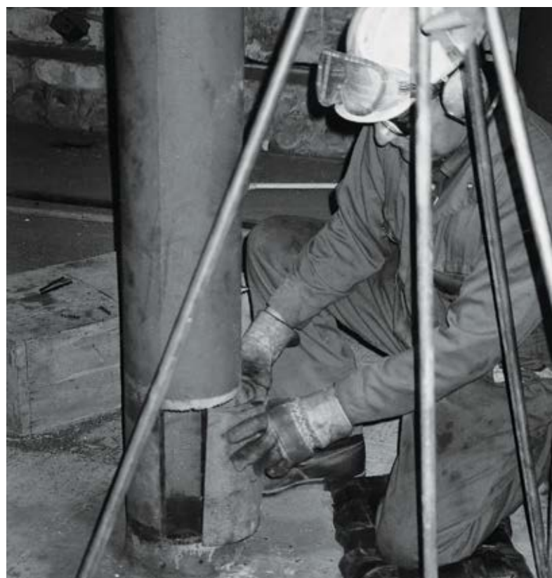
Above: Support column repair from beginning to end, using the Metallock process.
